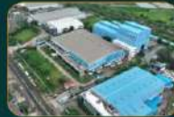
BHEL TRICHY BHARATH HEAVY ELECTRICALS LT.
